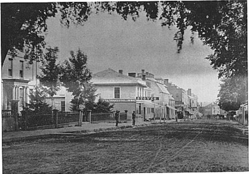
Tilton House ( above ), one of the few residences left on upper State Street, now sympathetically adapted to apartments. Residential upper State Street merges into the commercial ( below ). Building at left is the present Public Library in which Washington and Lafayette were once entertained. In later years, Newburyport's well-known eccentric, Lord Timothy Dexter, occupied the house for a time. Two rooms retain original paneling and fireplaces.
