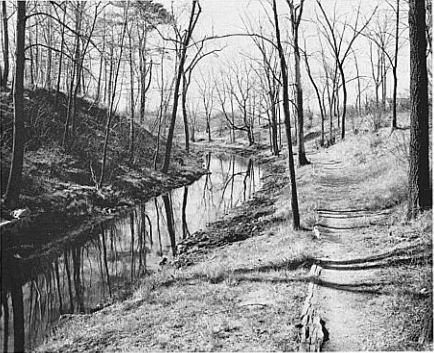
VIEW LOOKING SOUTH DOWN THE MIDDLESEX CANAL, SCHOOL STREET, NORTH WOBURN, MASSACHUSETTS
