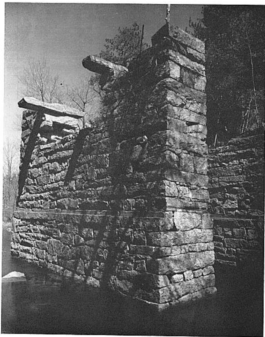
SHAWSHEEN AQUEDUCT, LOOKING NORTHEAST, MIDDLESEX CANAL, WILMINGTON—BILLERICA, MASSACHUSETTS
