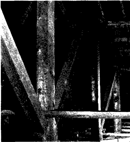
FIG. 4. KING POST (left) AND QUEEN POSTS (right), WEST CHURCH. (Photo by William W. Owens, Jr.)
