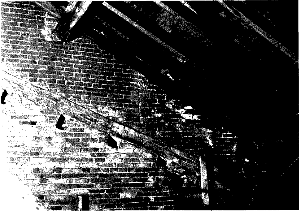
FIG. 3. INTERIOR FRONT WALL OF WEST CHURCH, ABOVE THE CEILING. Note the original roof line and purlin holes. (Photo by William W. Owens, Jr.)
