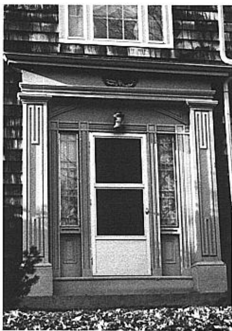
FIG. 6. DOOR OF THE PELETIAH P. PIERCE HOUSE, renovated c. 1834, at 1106 Massachusetts Avenue, East Lexington. (Photo by Elizabeth W. Reinhardt.)
