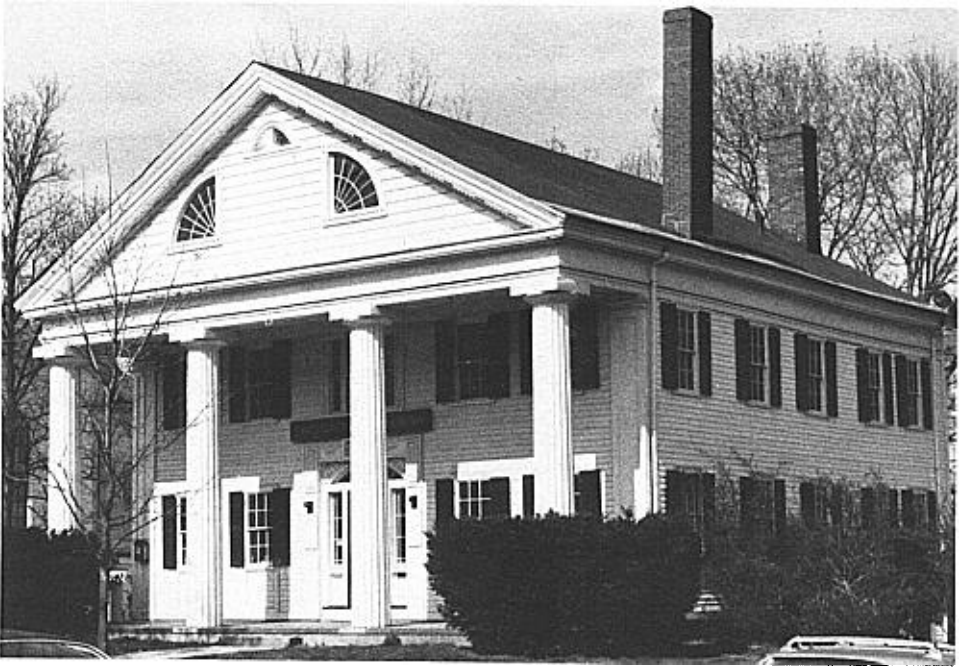
FIG. 1. THE STONE BUILDING, 715 Massachusetts Avenue, East Lexington, which now houses the East Lexington Branch Library. Originally designed as a lecture hall by Isaac Melvin, 1833. (Photo by Elizabeth W. Reinhardt.)
