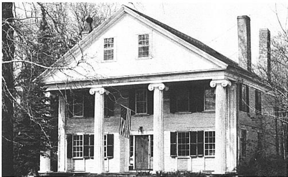
FIG. 11. AMBROSE MORELL HOUSE, 627 Massachusetts Avenue, East Lexington, built c. 1800, remodeled 1839. Note the brick side wall at right, with a stringcourse between the first and second stories. (Photo by Elizabeth W. Reinhardt.)
