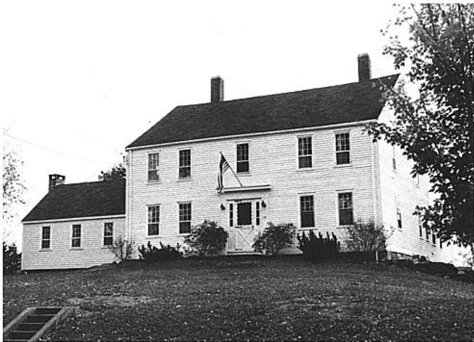
FIG. 1. ENOCH NOYES'S HOUSE, 127 Main Street, West Newbury. (Photograph by the author.)
