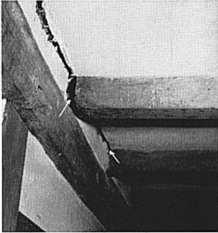
FIG. 2. INNER FACE OF END GIRT SHOWN IN FIG. 1 WITH FLOOR JOISTS AND CEILING ABOVE, PLASTERED BETWEEN THE JOISTS
