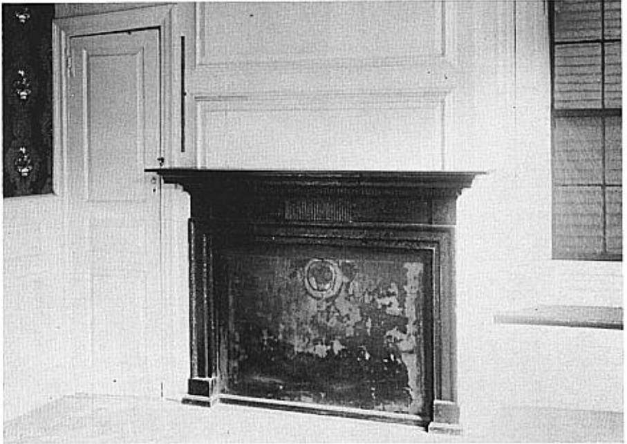
DERBY HOUSE, SALEM, MASSACHUSETTS. FIREPLACE IN THE EAST FRONT ROOM, BEFORE RESTORATION
